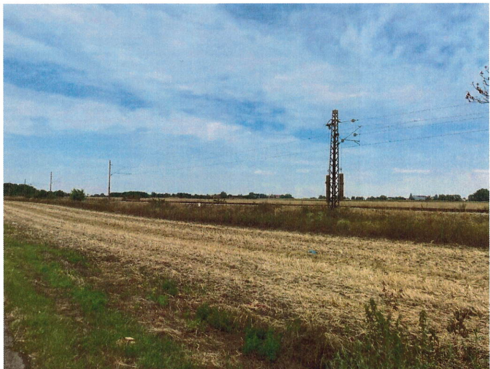
Existing railway-track across the access road
